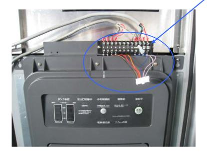
Loosen two screws, which is locating on left figure, and remove the terminal block cover.
