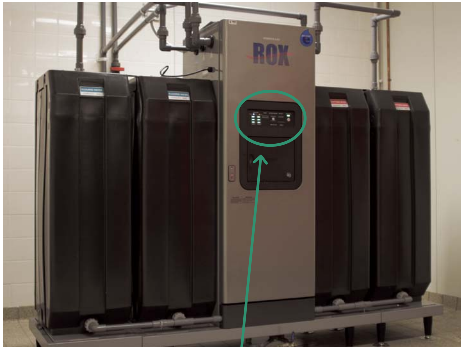
EWATER REMOTE CONTROL IS A REPLICA OF THE OPERATING PANEL ON THE BASE PLANT
